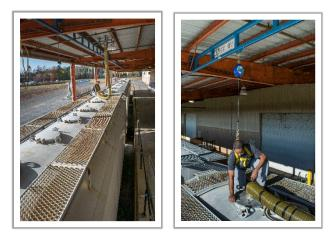
A Gorbel Tether Track Monorail system was chosen as the best option and by notching the canopy beams, the track was able to be raised up into the girder underneath. The notched areas were then reinforced with angle iron that was bolted into place. This allowed for the proper height requirements to be met. The Tether Track Fall Protection System gave the on-site safety manager reassurance that the employees are kept safe when they are on top of the rail cars.
